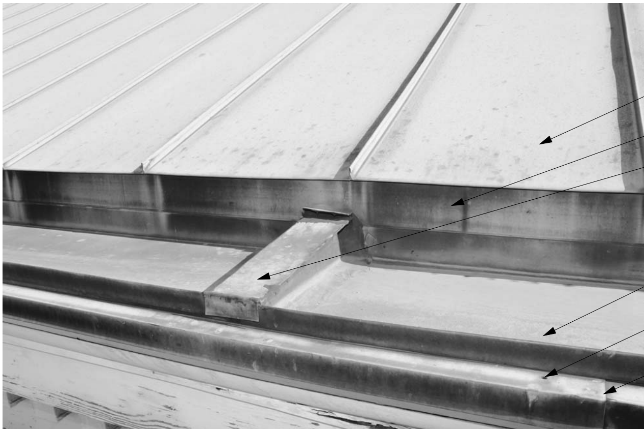
3 EXISTING CONDITIONS- DETAIL OF GUTTER EXPANSION JOINT N.T.S.
