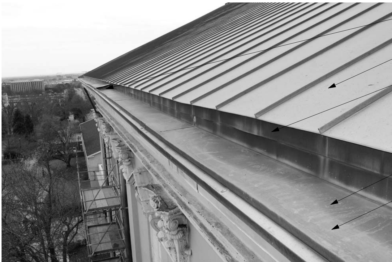
1 EXISTING CONDITIONS- GUTTER EXPANSION JOINT @ EAST ELEVATION N.T.S.
