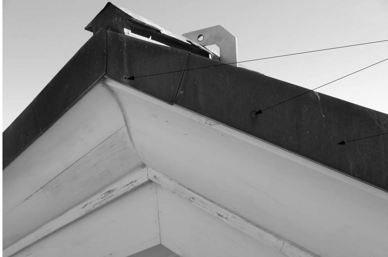
2 EXISTING CONDITIONS- NORTH ELEVATION ROOF FLASHING N.T.S.
