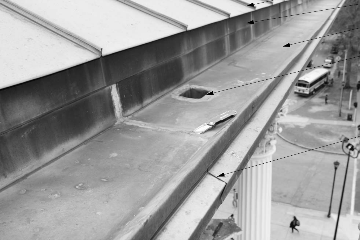
2 EXISTING CONDITIONS- GUTTER DOWNSPOUT INLET N.T.S.
