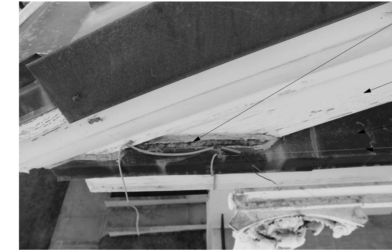
2 EXISTING CONDITIONS- PEDIMENT FLASHING DETAIL @ NORTH ELEVATION, NE CORNER N.T.S.
