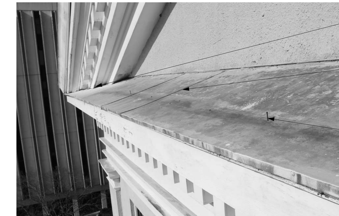
4 EXISTING CONDITIONS- PEDIMENT FLASHING DETAIL @ SOUTH ELEVATION N.T.S.
