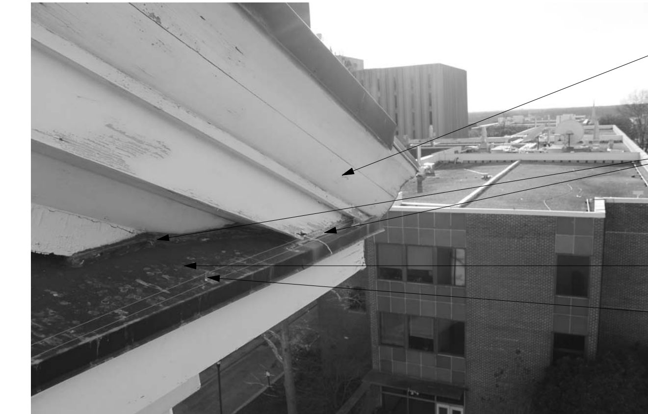
3 EXISTING CONDITIONS- PEDIMENT FLASHING DETAIL @ NORTH ELEVATION, NW CORNER N.T.S.
