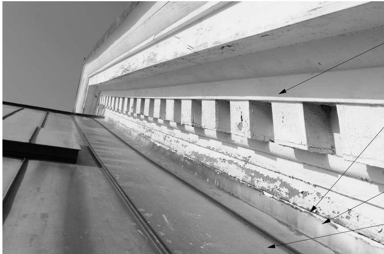
3 EXISTING CONDITIONS- SOUTH ELEVATION ROOF FLASHING N.T.S.
