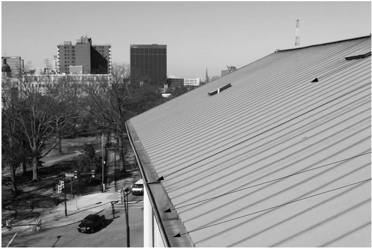
2 EXISTING CONDITIONS- GUTTER EXPANSION JOINT @ WEST ELEVATION N.T.S.
